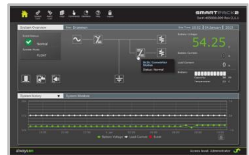
STATUS OF DC/DC CONVERTERS IN SMARTPACK2 WEB
